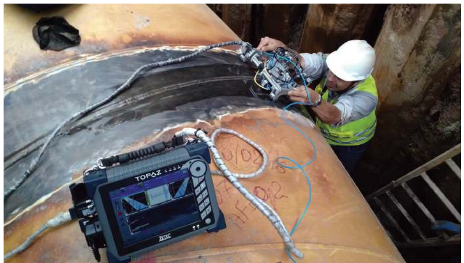
Fig. 3 — Improved portability and processing have brought PAUT weld inspections to locations that were once considered out of reach. (Photo courtesy of Zetec, Empresas Concremat.)
